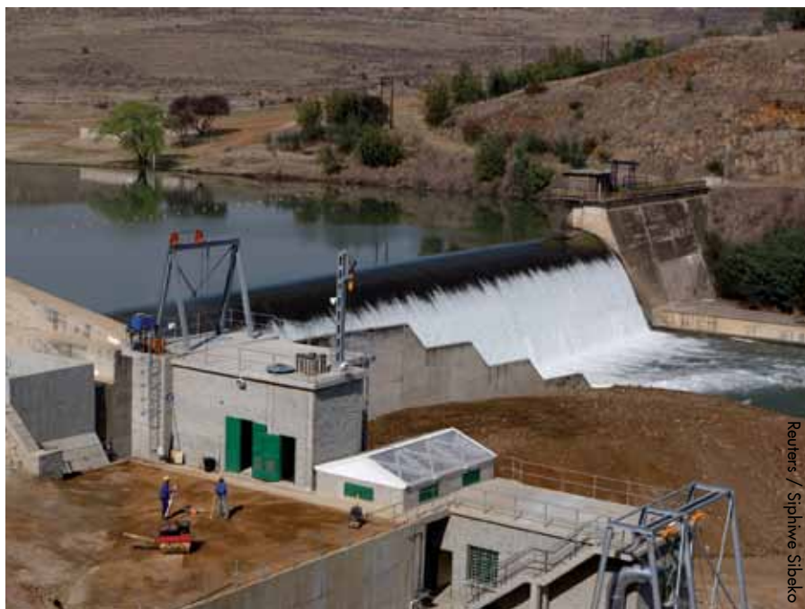
A mini hydro-electric plant near Bethlehem in South Africa
